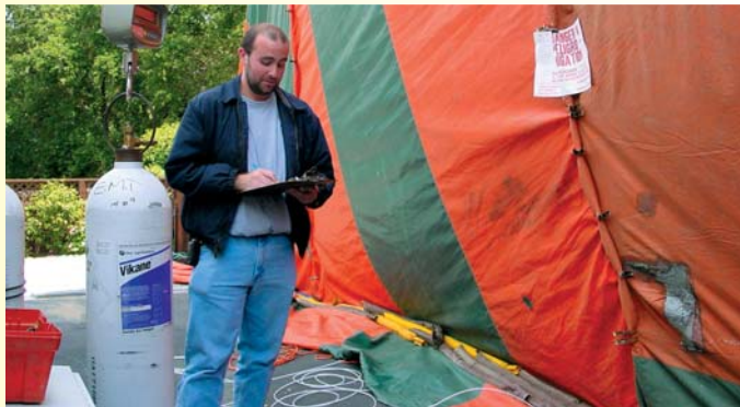
Monitoring a structural termite fumigation
