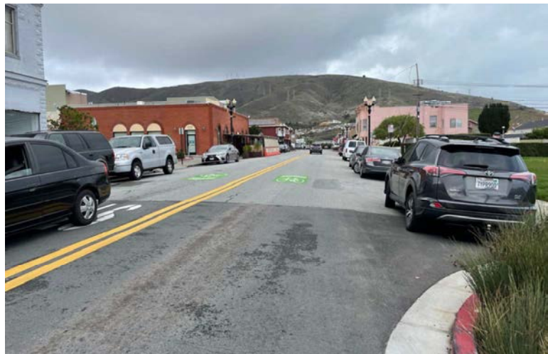
14 - Intersection of Linden & Pine Avenues – Direction is North
