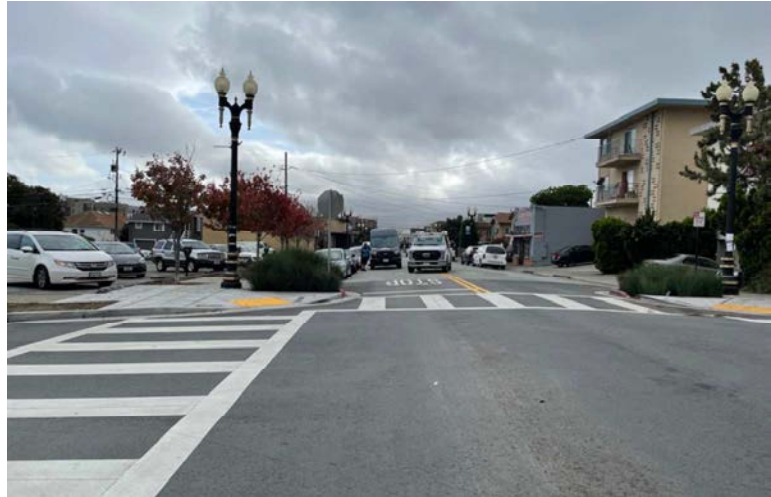
13 - Intersection of Linden & Pine Avenues – Direction is South
