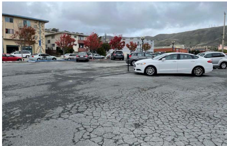
2 - 616 Linden Avenue – Southeast Corner – Direction is Northwest
