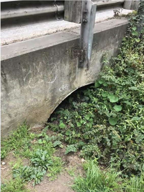
Photograph 17: Culvert (CWUS-4) for unnamed intermittent creek west of SR 1
