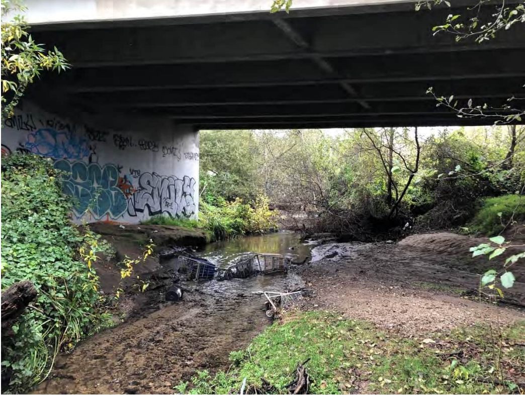
Photograph 3: Pilarcitos Creek (OWUS-1) under the SR 1 northbound bridge.
