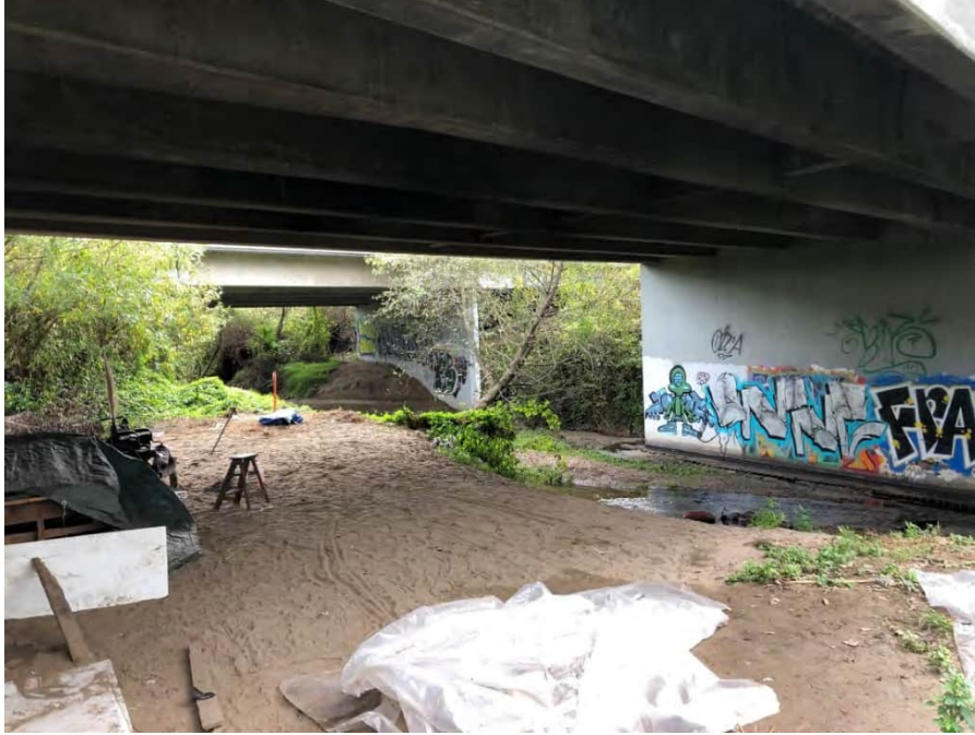
Photograph 1: Pilarcitos Creek (OWUS-1) under SR 1 southbound bridge.
