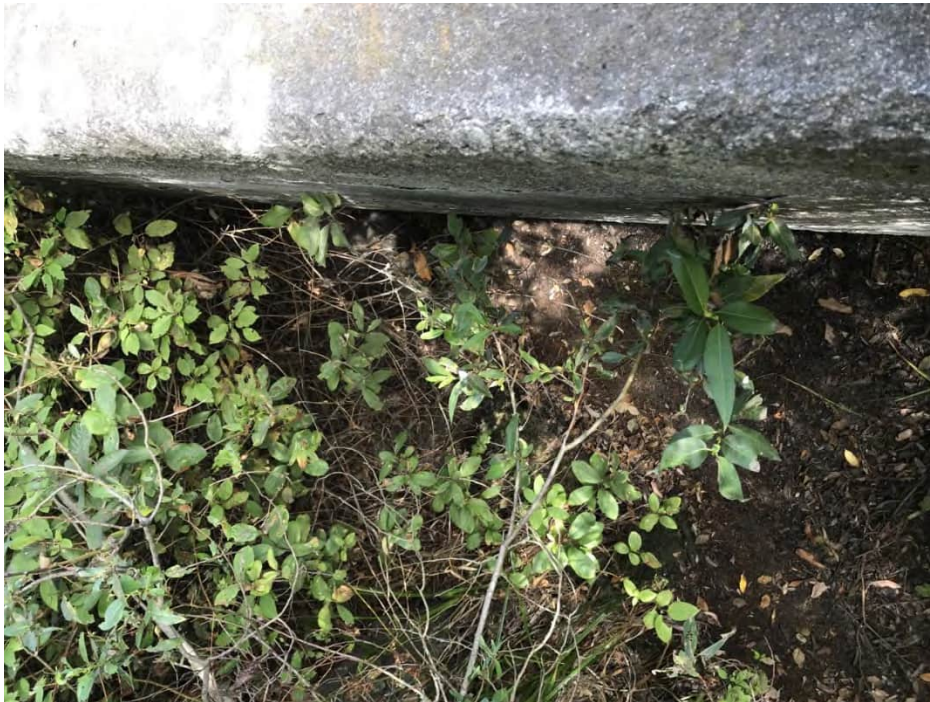
Photograph 32: Streambed of Denniston Creek (OWUS-9b) next to the culvert (CWUS-7) headwall.
