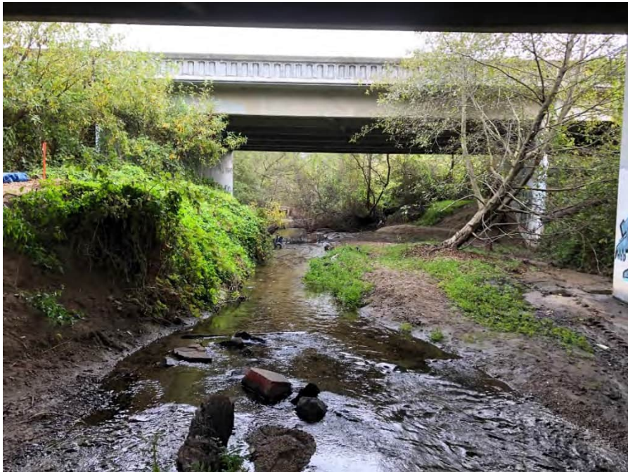
Photograph 2: Pilarcitos Creek (OWUS-1) facing the SR 1 northbound bridge.
